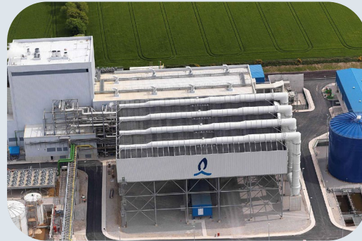
Whitegate 445MW CCGT
