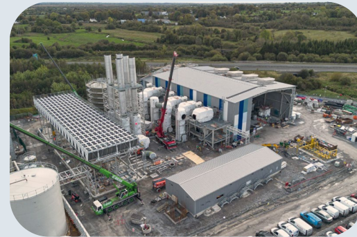
Dublin & Athlone 2 x 100MW reciprocating engines
